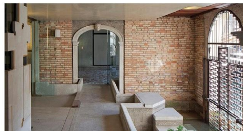
Floodable entryway with stairs that lead to an elevated lobby at the Querini Stampalia in Venice, Italy. Photo: Architectours / "The renovation of the Fondazione Querini Stampalia is a great example of how Master Carlo Scarpa integrated the new with the old"
